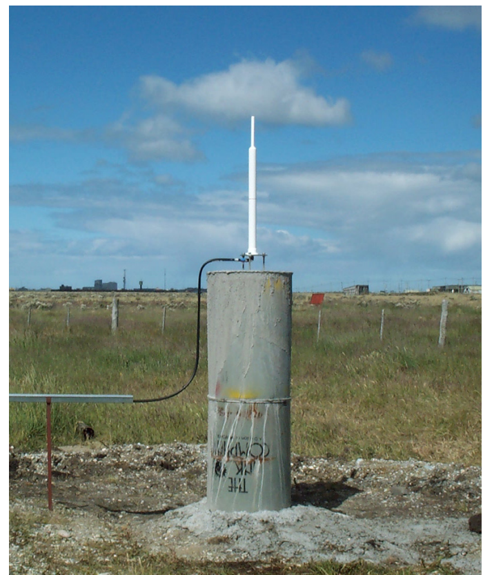
Renovation (2001): deeply anchored concrete pillar, A4 stainless steel plate
