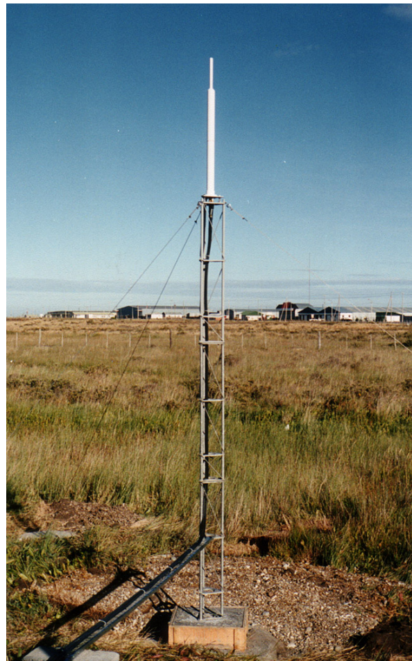
First upgrade (1995): Starec antenna, good quality guying, mm-level centring and verticality
