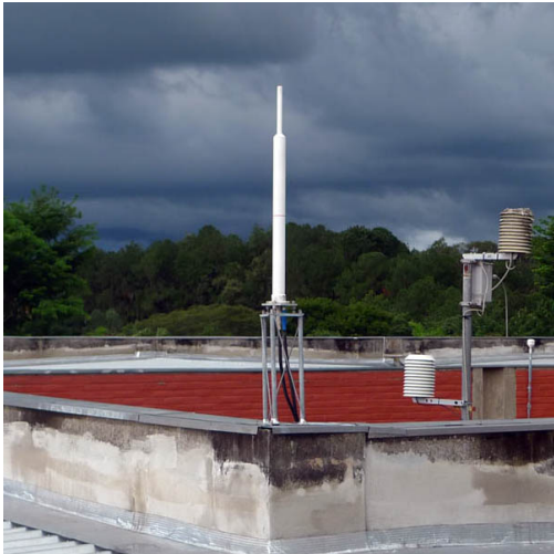
Type I (29%): steel tower on load-bearing wall of building
