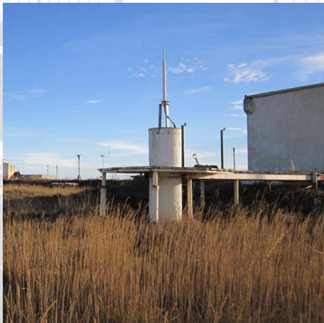
Rio Grande, Argentina ( RISC ). Restarted after 2-yr outage: Aug. 28, 2018.
